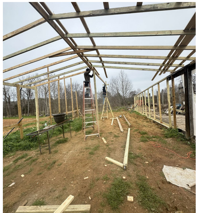
Greenhouse frame construction
